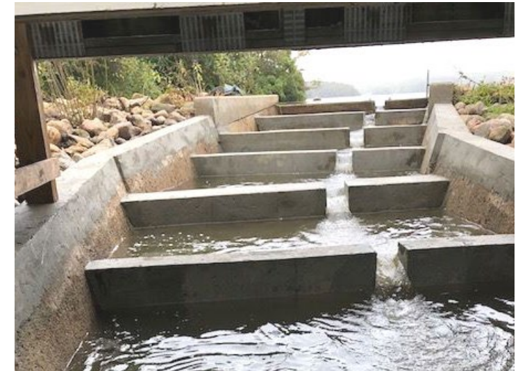
Indian Lake fish ladder completed.
